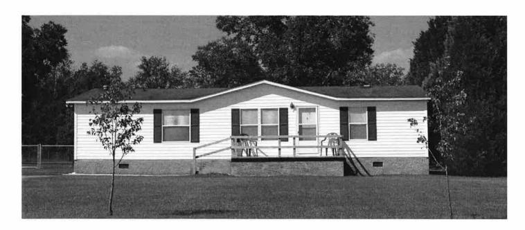
Manufactured homes are transportable structures that are fixed to a chassis and specifically designed to be towed to a residential site. They are not the same as modular or prefabricated homes, which are factory built and then towed in sections to be installed at a permanent location.
